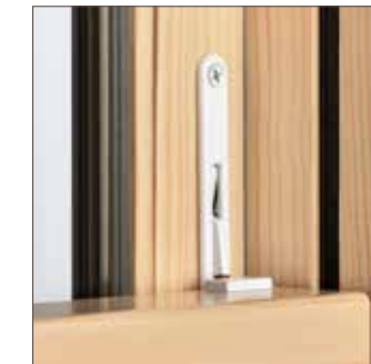
Push both WOCDs in to open the sash more than 4 inches
